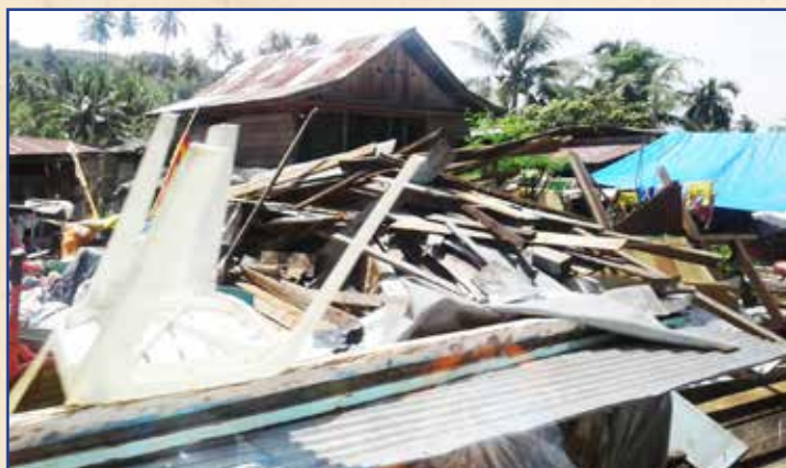
Devastation of houses by earthquake
